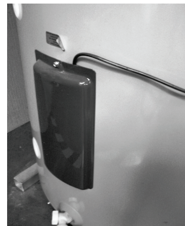
Figure 17 - Lower Tank Sensor
