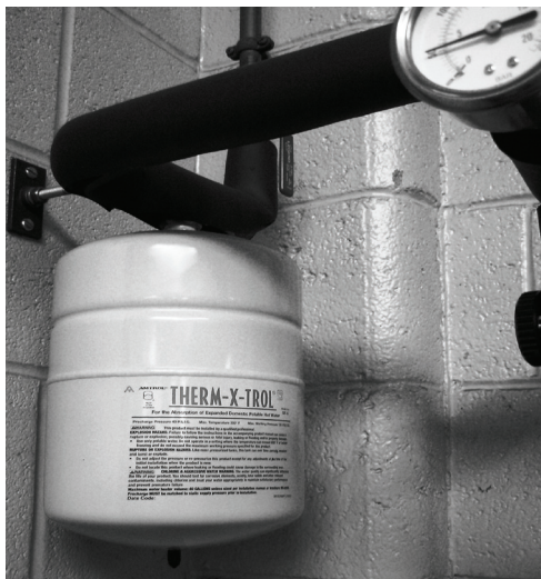
Figure 14 - Expansion Tank
